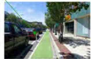
Parking-protected bike lane with paint to define lane boundaries
