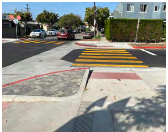
High visibility crosswalk. Crossing installation in Culver City, CA. Wide continental crosswalk striping and directional ramps make this design very comfortable for pedestrians.
