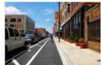
Bike lane with cross-hatched buffer adjacent to travel lane with flexible bollards
