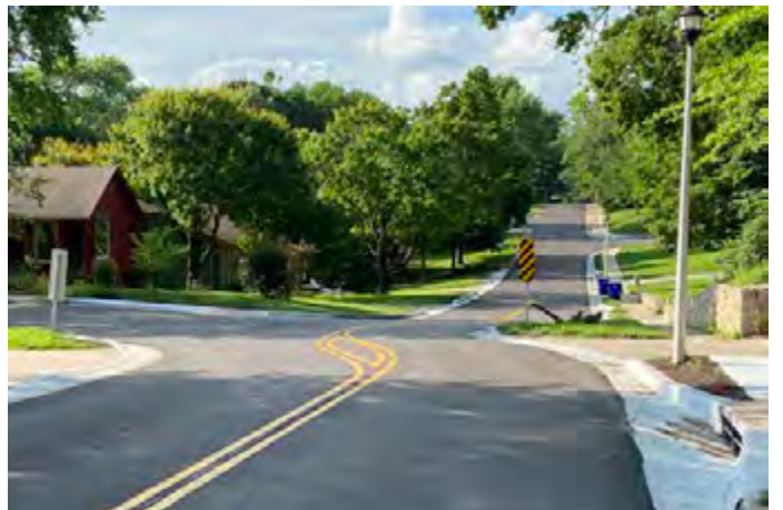
Chicanes or street realignment at specific locations. Goodman Street in Merriam, KS)
