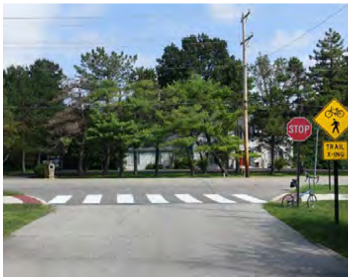
High visibility crosswalk and trail advisory sign, Clayton Road, Saint Louis County, MO
