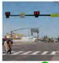
Hybrid (HAWK) beacons If it increases compliance, RFBs on 30 Dr. How do not work here.
