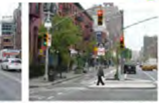
Parking-protected bike lane with raised curb at corners to define parking lane and provide pedestrian protection (inter-wall)
