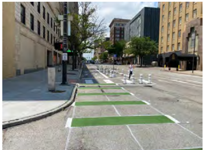
Cycle track. This installation is designed as a pilot project using flexible delineators. Note the "continental style" crossing markings in green..
