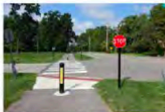
Sidepath with grass separation from roadway and clear driveway and street crossing definition
