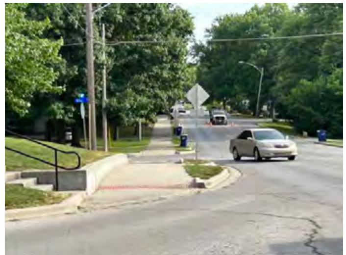
Shared Use Sidepath. Nall Avenue path accommodates travel in both directions. Warning signs for motorists and high visibility crosswalks at street crossings will add to the safety of these facilities
